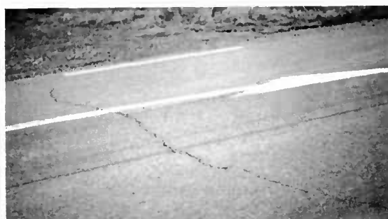
Fissure transversale
